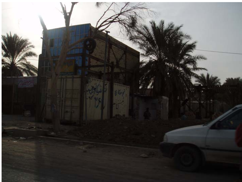
Picture 4. North edge of industrial part of city, next to residential area. Only surviving building on block. Collapsed buildings were made of standard brick. Flat terrain. 10-30 years old.
