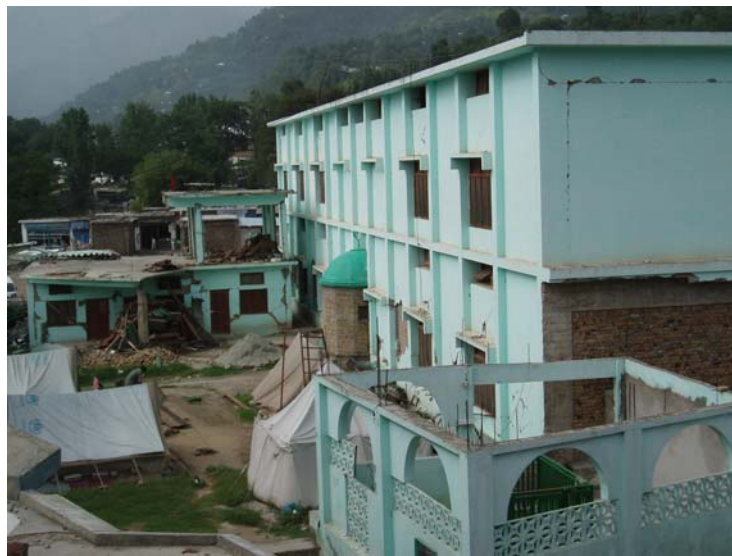
Picture 6. Eastern edge of residential area near the mountains. Flat terrain. All blue buildings built by same company with similar methods. Minimal structural damage, some small wall collapse. 10-20 years old.
